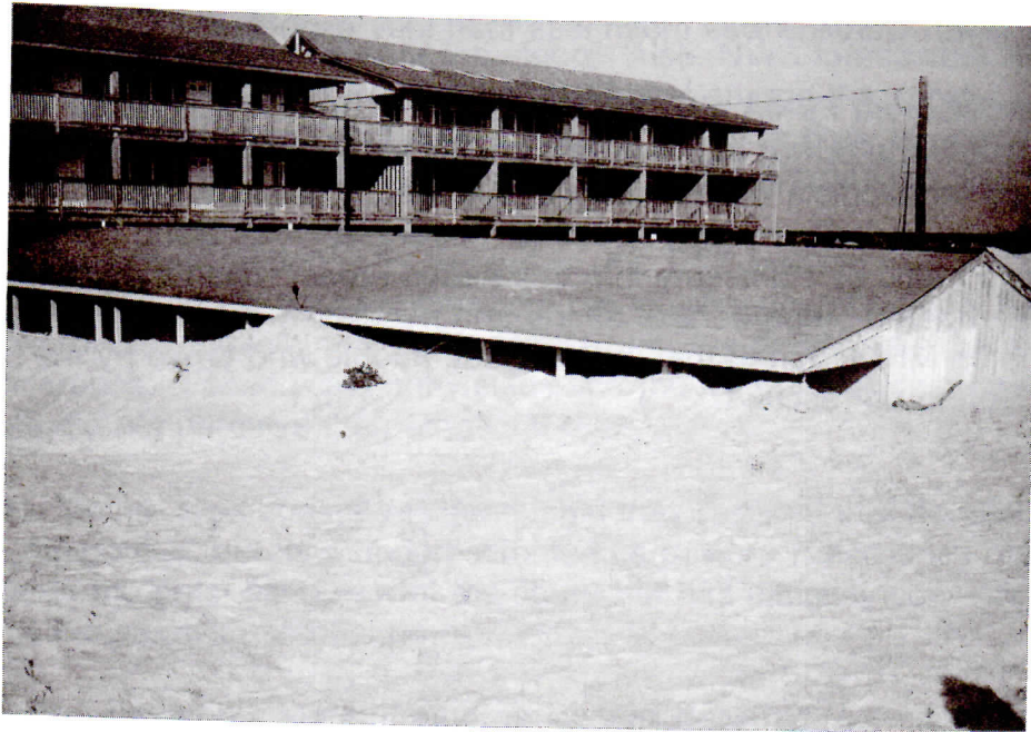
Figure 28. Sand buried motel in Buxton, North Carolina. Photo courtesy of Mark Koehn.
