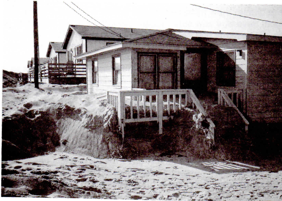
Figure 29. Sand buried beach house in Buxton, North Carolina. Photo courtesy of Mark Koehn.
